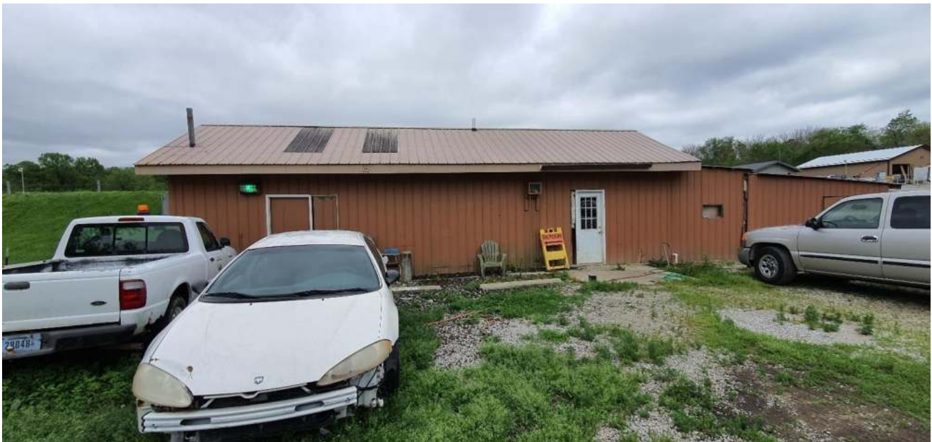
Figure 3-10 - Chemical Storage Building
