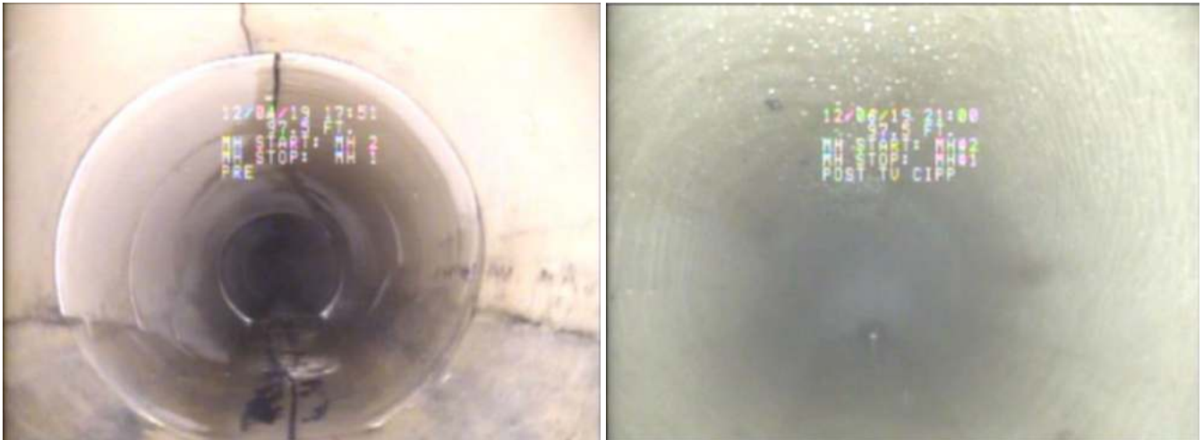
Figure 5-1- CIPP Lining Example Installation
