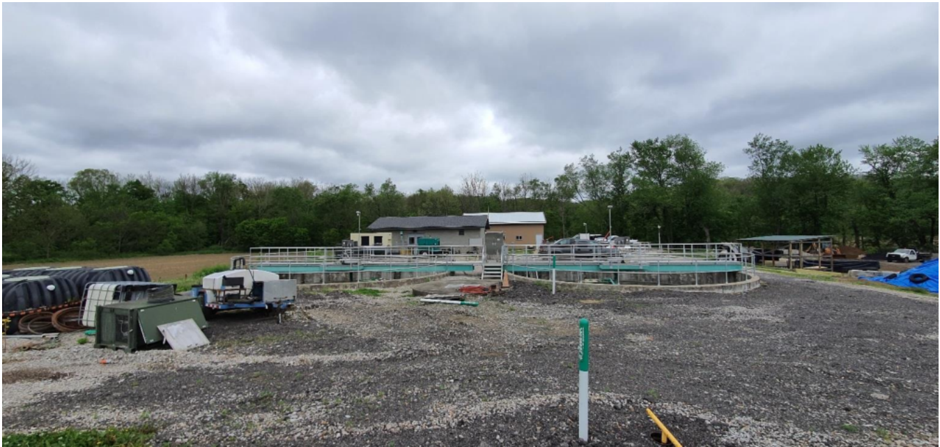
Figure 3-7 - Secondary Clarifiers
