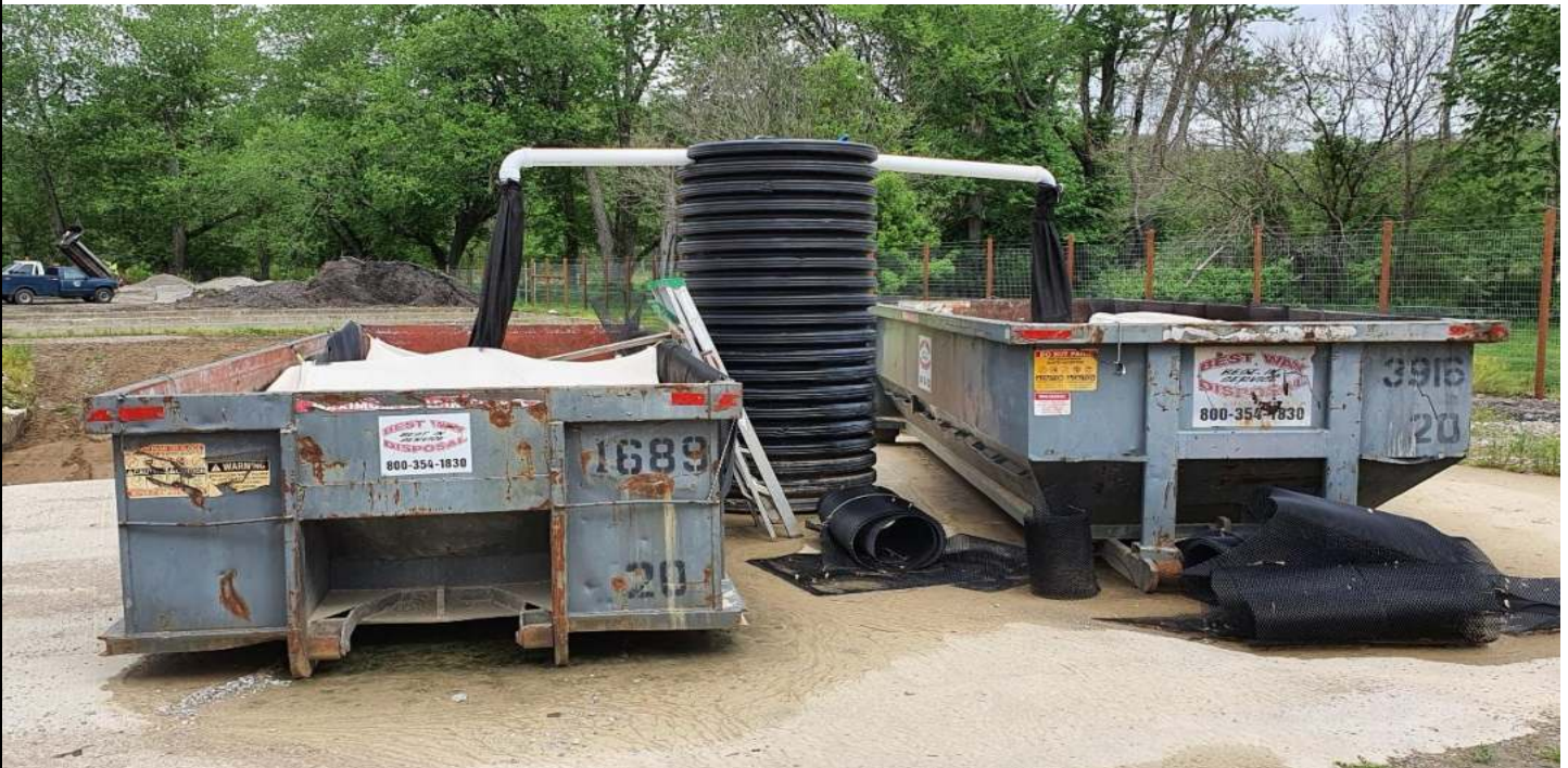
Temporary Geosynthetic Sludge Dewatering Bag System
