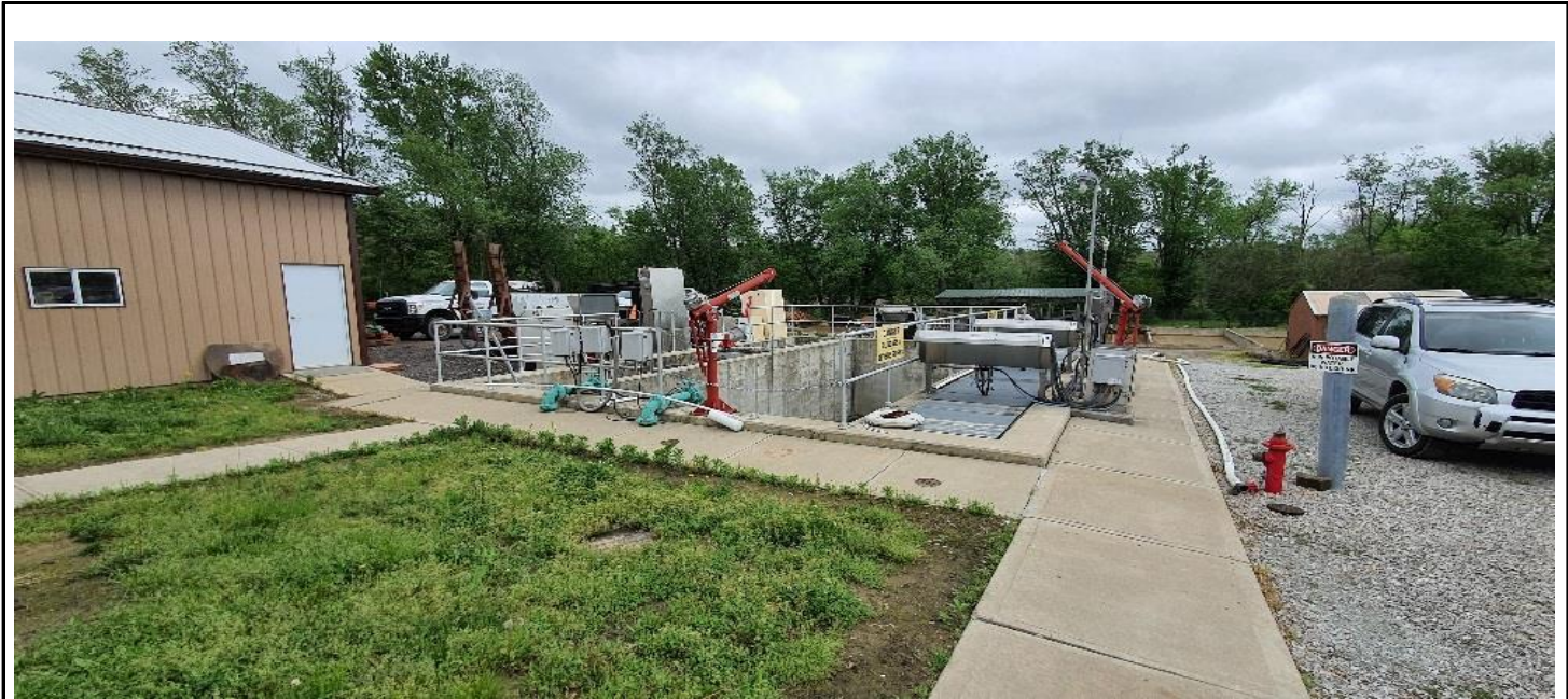
Disinfection & Post Aeration Structure
