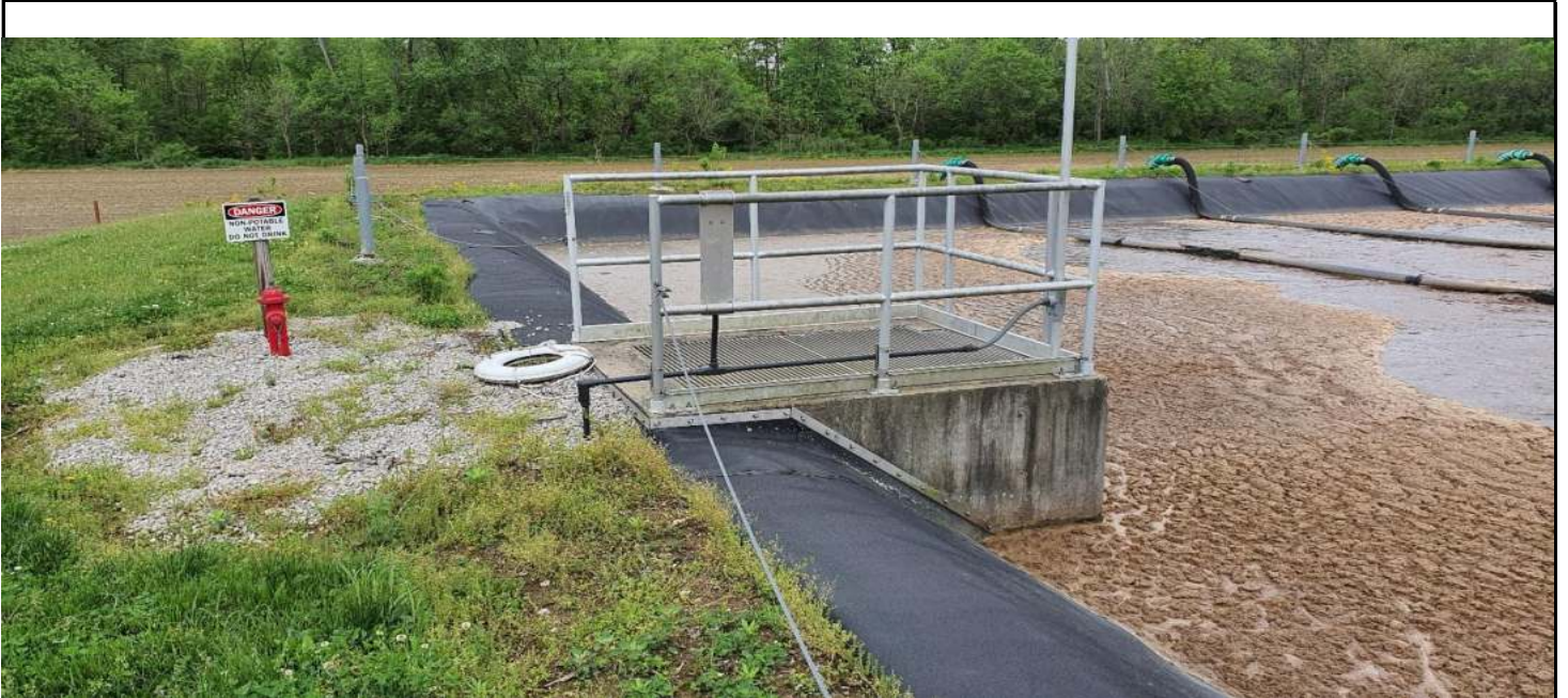
Aeration Lagoon - Influent Structure
