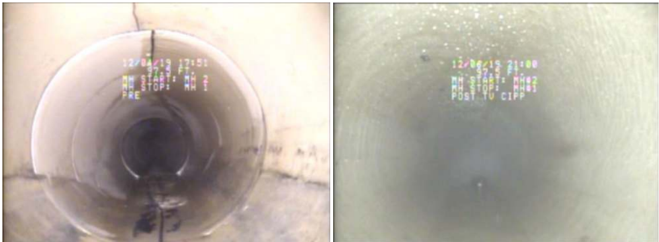
Figure 5-1- CIPP Lining Example Installation
