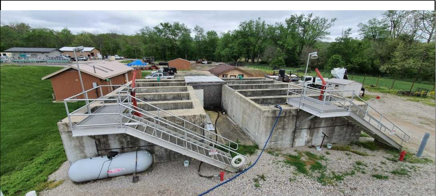
Aerobic Digesters
