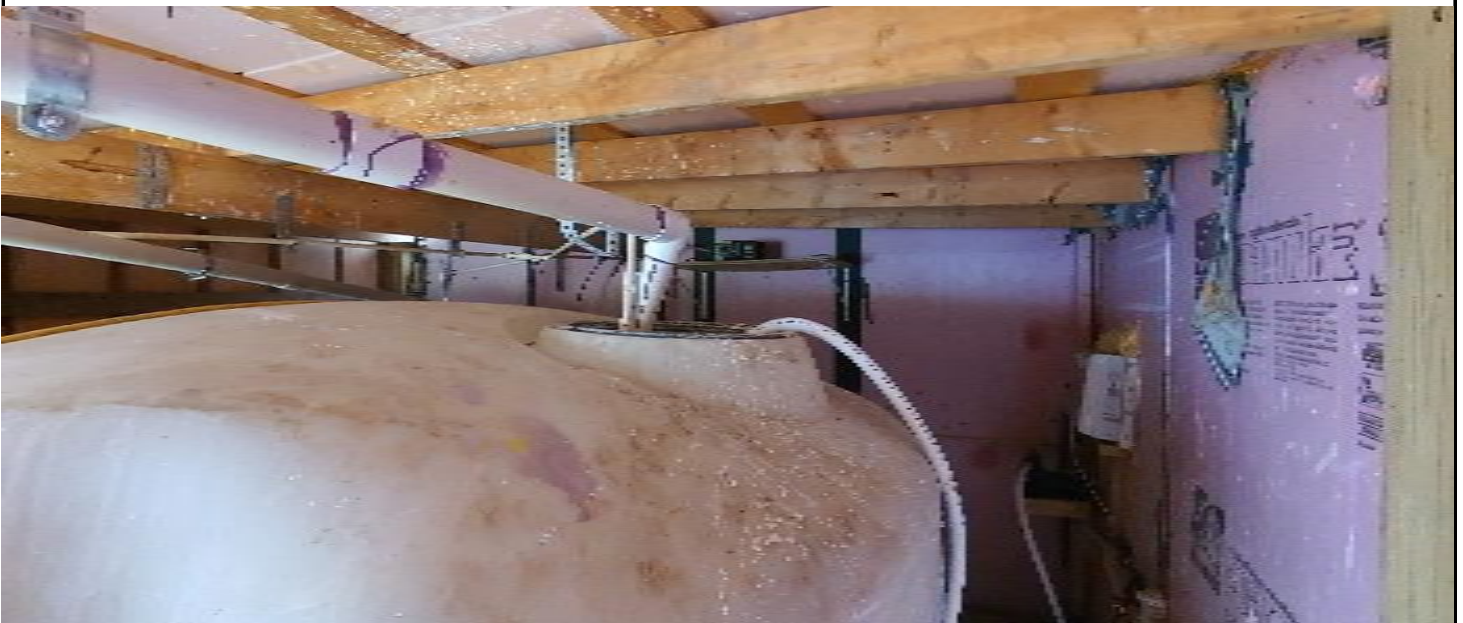
Chemical Storage Building - Chemical Room
