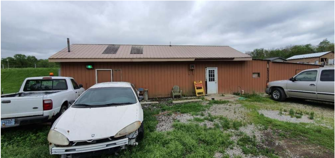
Figure 3-10 - Chemical Storage Building
