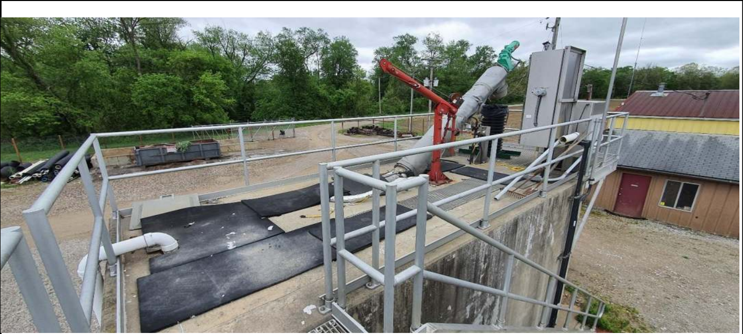
Headworks Mechanical Fine Screen, Hoist, and Conveyer
