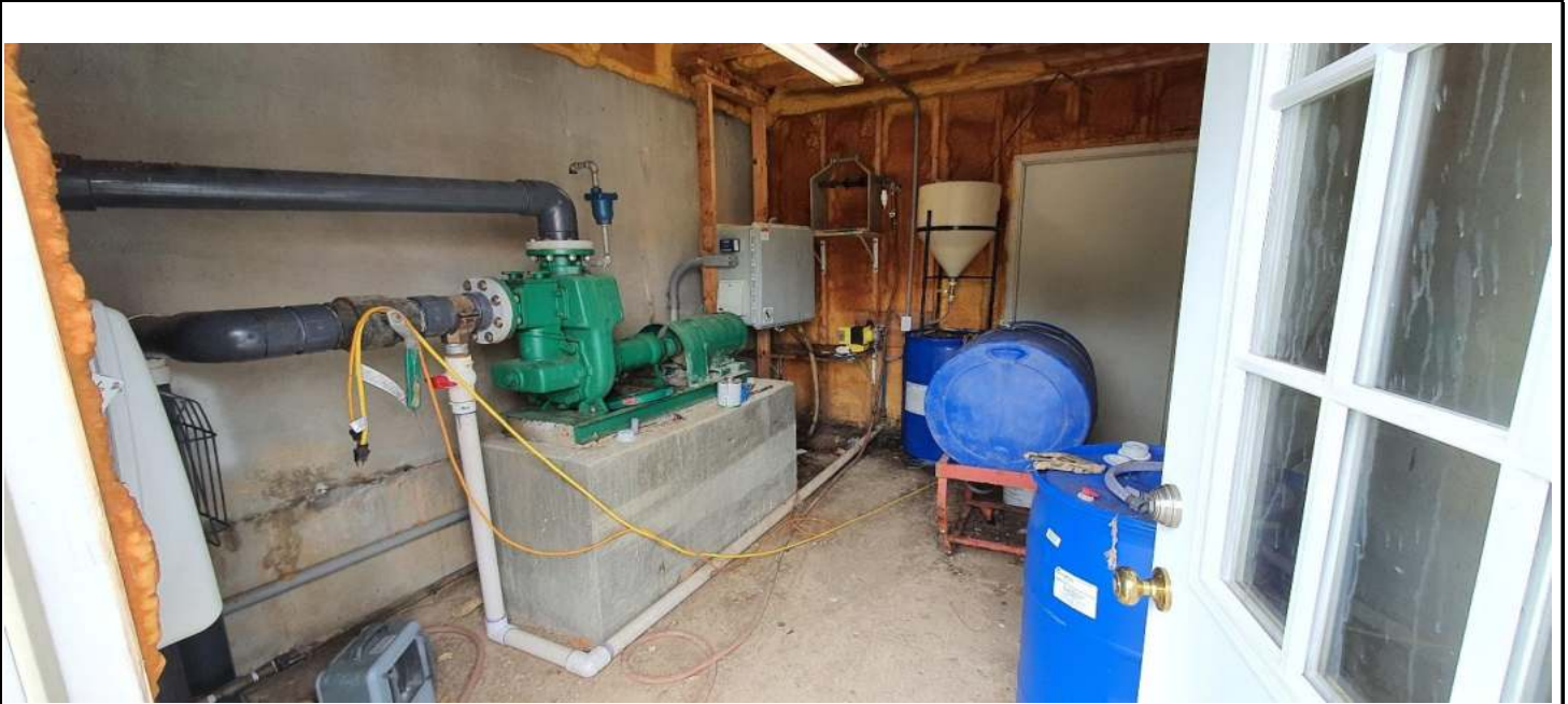
Sludge Pump Building
