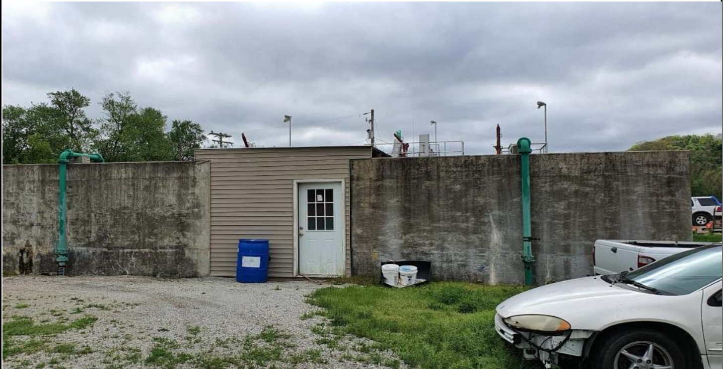
Sludge Pump Building
