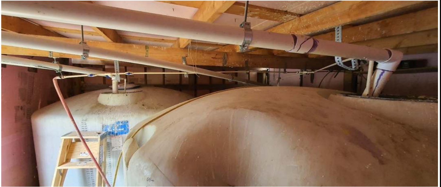
Chemical Storage Building - Chemical Room
