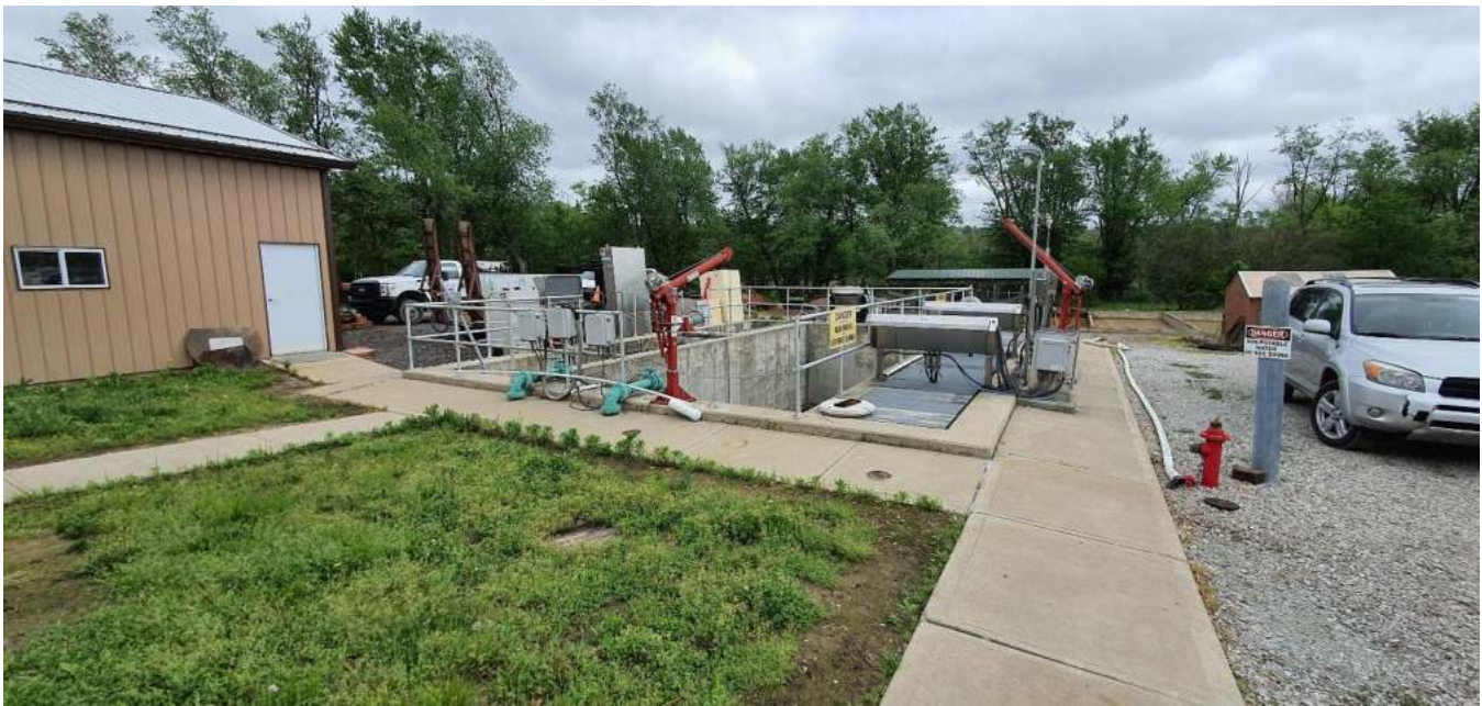
Figure 3-8 - Disinfection & Post Aeration Structure
