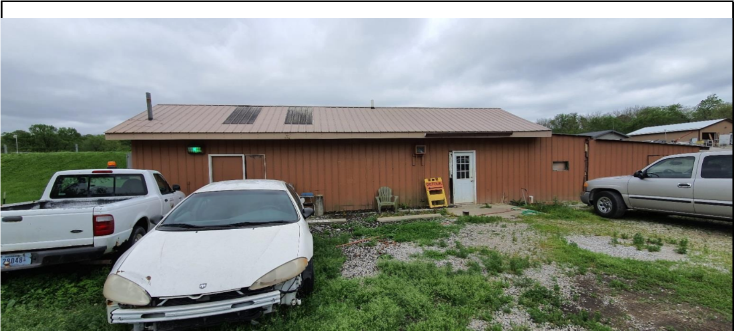
Chemical Storage Building
