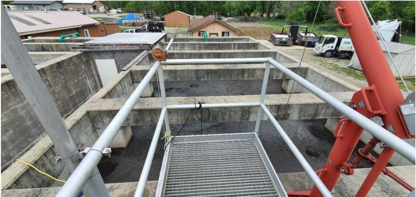
Figure 3-11- Aerobic Digester Tankage
